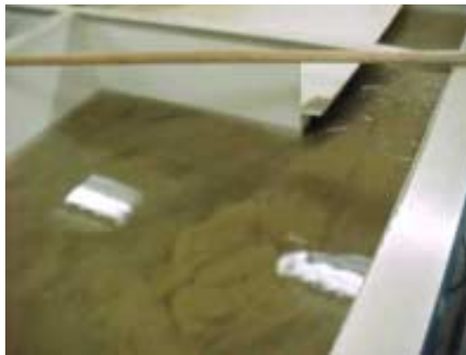
Figure 2-9 Sand filter backwashing
