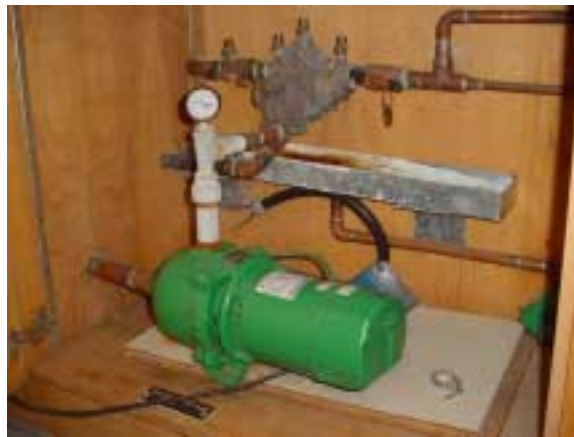
Figure 3-1 Centrifugal pump
